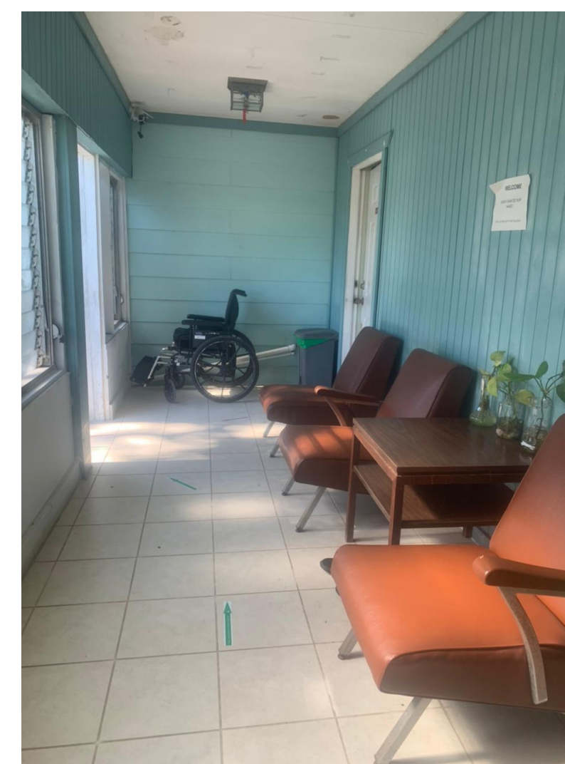
Image 3. Waiting area entrance after renovations
