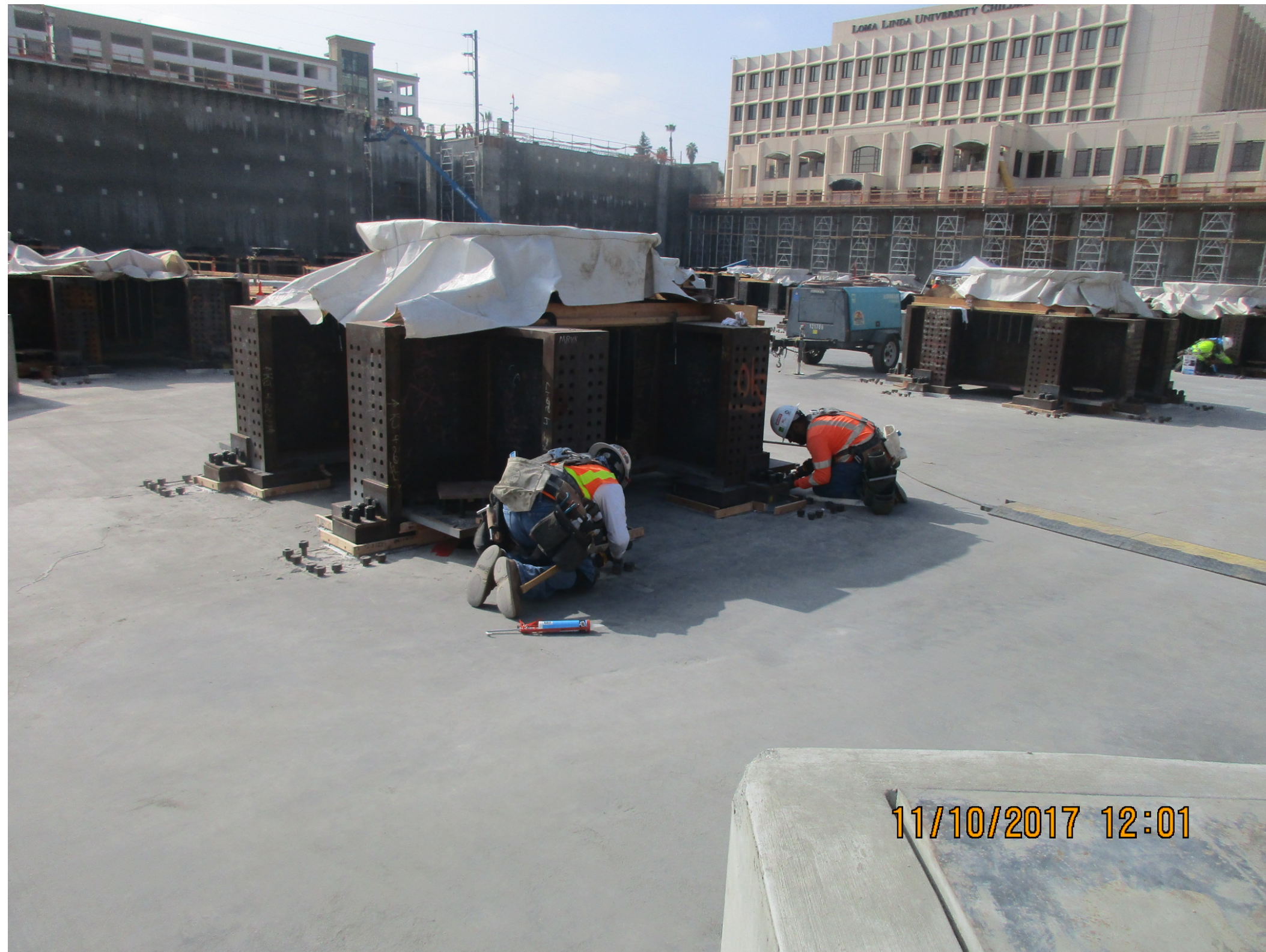
Grouting Pedestals to the Slab
