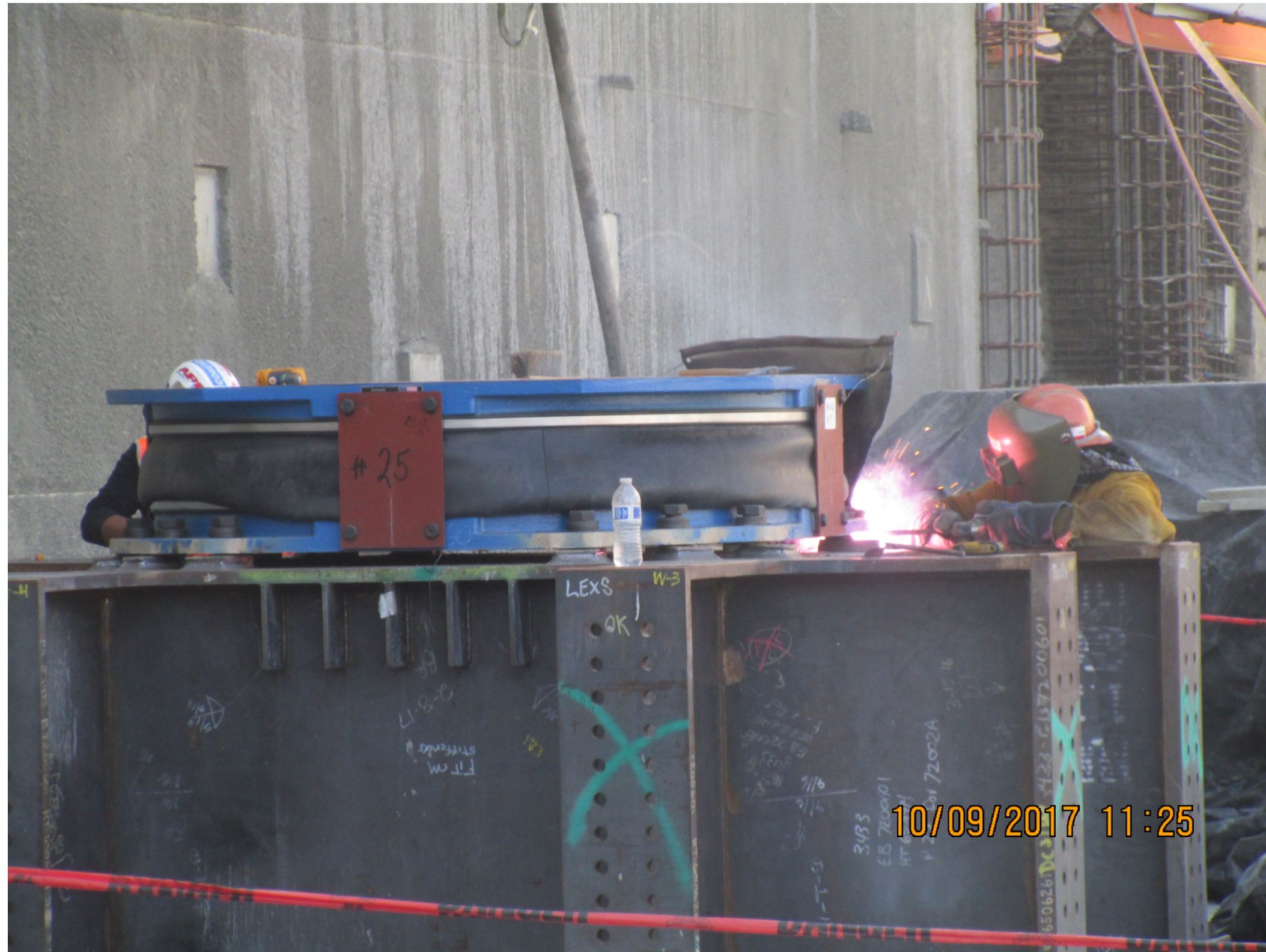
Preparing Isolators for Grouting
